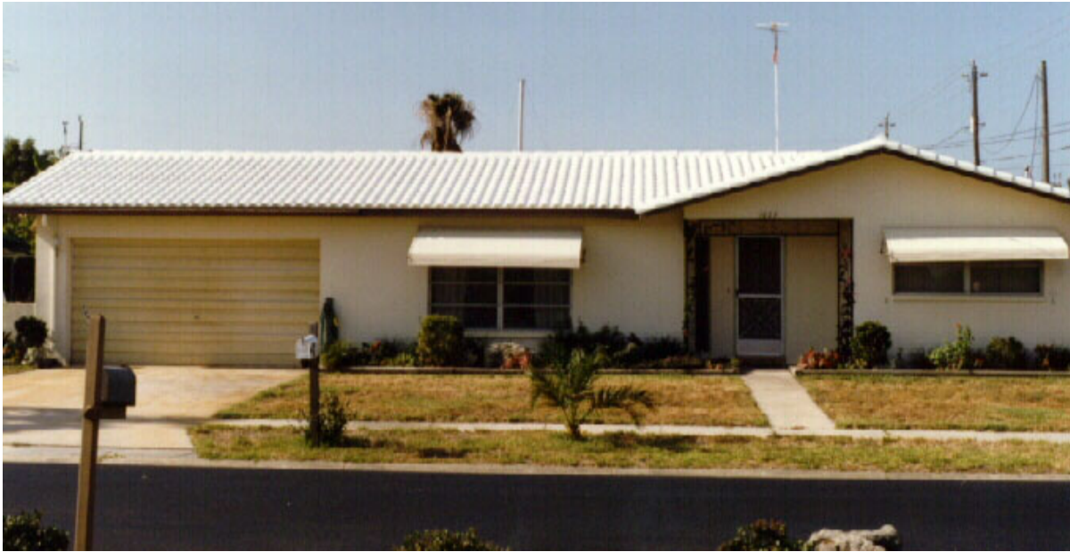
Figure A2. Site #5 after coating.
