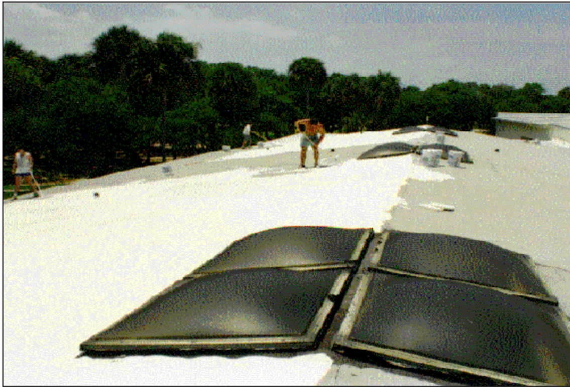
Figure 12. First of three coats of white acrylic elastomeric is applied to school roof on May 9, 1995.
