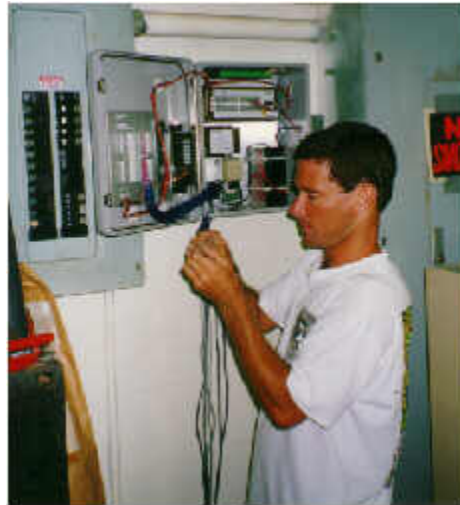
Figure 6. John Sherwin wires in data logger to collect 15-minute data on weather, building thermal conditions, and cooling system electric power.
