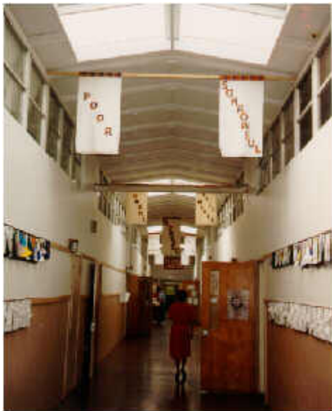
Figure 2. Central unconditioned hallway.
