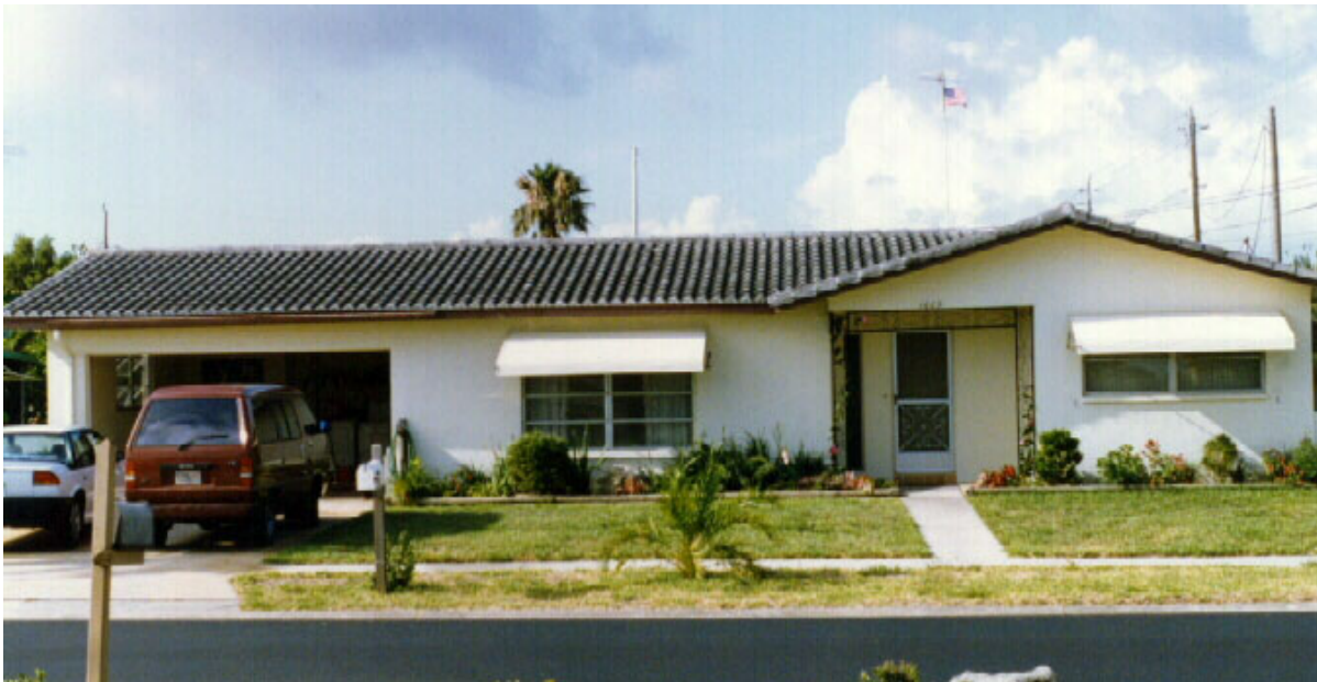
Figure A1. Site #5 before coating.
